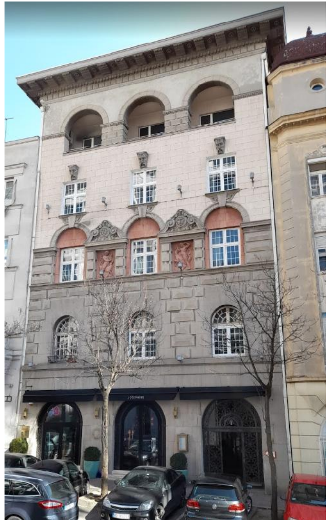
Picture 23 - Josif Šojat Building, today
