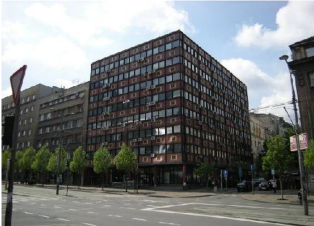
Picture 28a - Social security building
