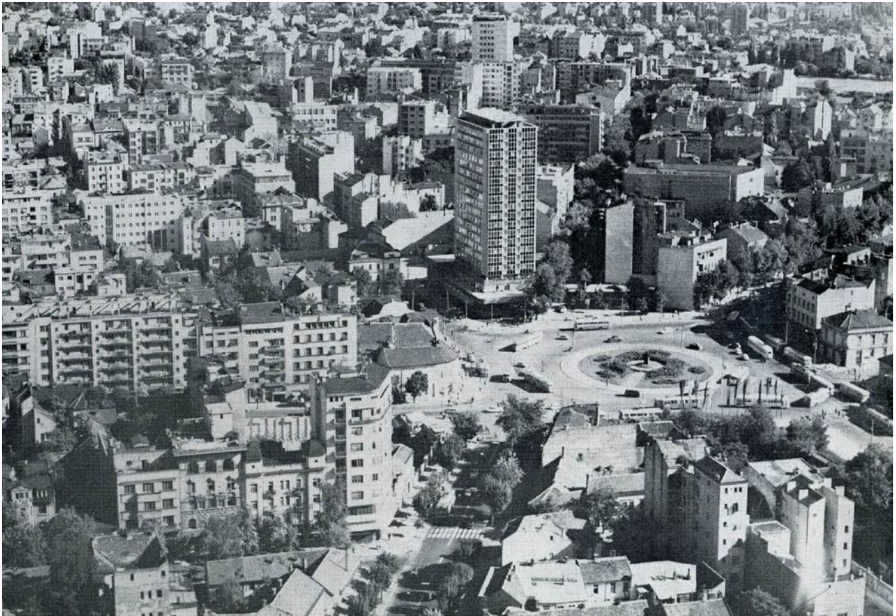
Picture 18 - aerial shot of Slavija from Svetozar Markovic to Vracar, 60s of the XX century
