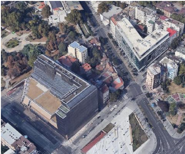
Figure 12 - view of the block towards Manjez
